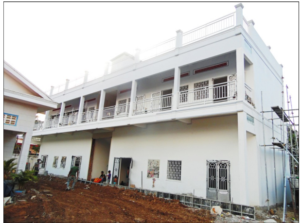
New Bible School Building is Nearly Finished
