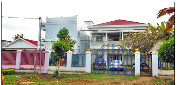
Left to Right: Faith Bible Church, New Bible School Building, Renovated Children's Home Building
