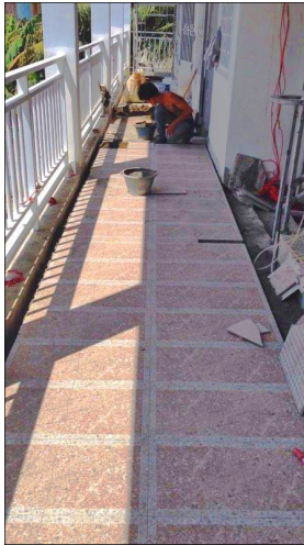
Upstairs Walkway Being Tiled
